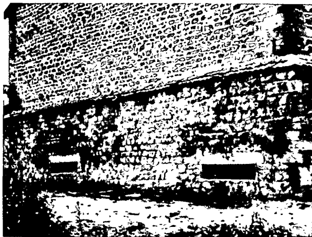
Figure 19. Typical firing ports and observation slits in wall of masonry building.
