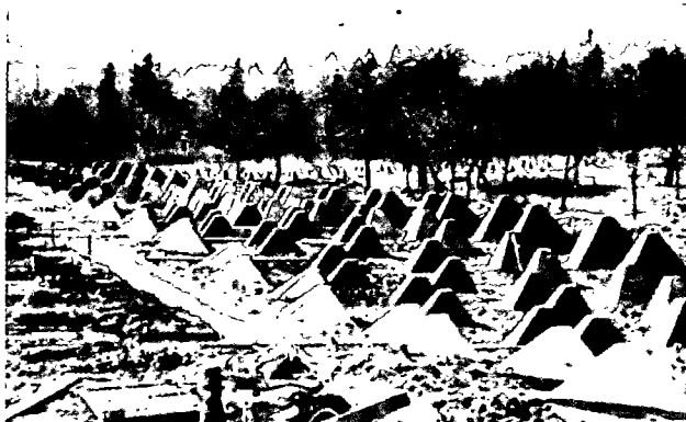
Figure 4. Dragon's teeth, showing five double rows.
